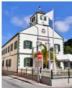
the Courthouse, built in 1793 following the founding of Philipsburg in 1763
