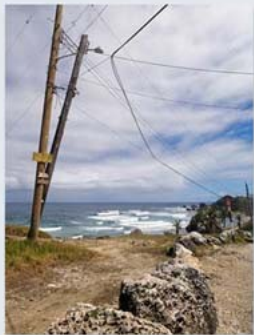
electrical power lines everywhere
