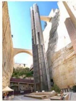
The Upper Barrakka lifts opened in 2012, linking the Grand Harbour to the Upper Barrakka Gardens and the city centre. The earlier lift was dismantled in 1983, having operated since 1905. The two lifts, which travel 58 metres can each carry 21 people, the journey taking twenty-five seconds.
