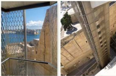
The Upper Barrakka lifts opened in 2012, linking the Grand Harbour to the Upper Barrakka Gardens and the city centre. The earlier lift was dismantled in 1983, having operated since 1905. The two lifts, which travel 58 metres can each carry 21 people, the journey taking twenty-five seconds.
